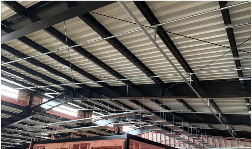
COUNTIES POWER OFFICES-AUCKLAND
